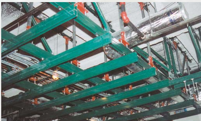
Multi-rail support system with Telespar drops.
