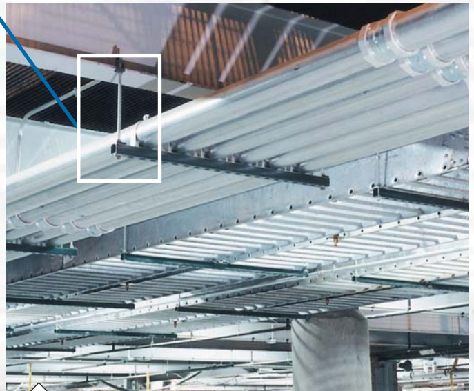
Beam clamp accepts standard threaded rod.
