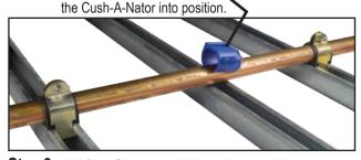
**Step 3:** Add Pipe Clamps and tighten the assembly.
