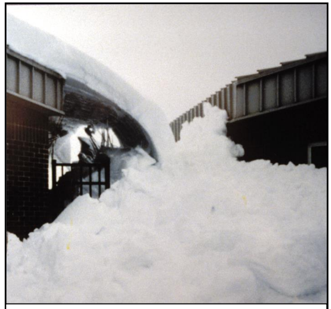
Figure 5: Sudden release of roof snow
