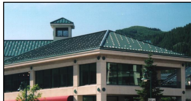
Figure 8B: “Cleat” type snowguard system
