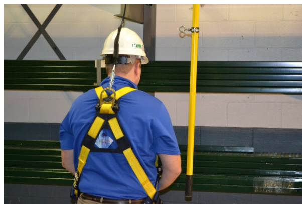
Figure 19 - Connect Snaphook to Harness Anchor Rated for 420 Pound Capacity Entire System Rated for 310 Pound Capacity
